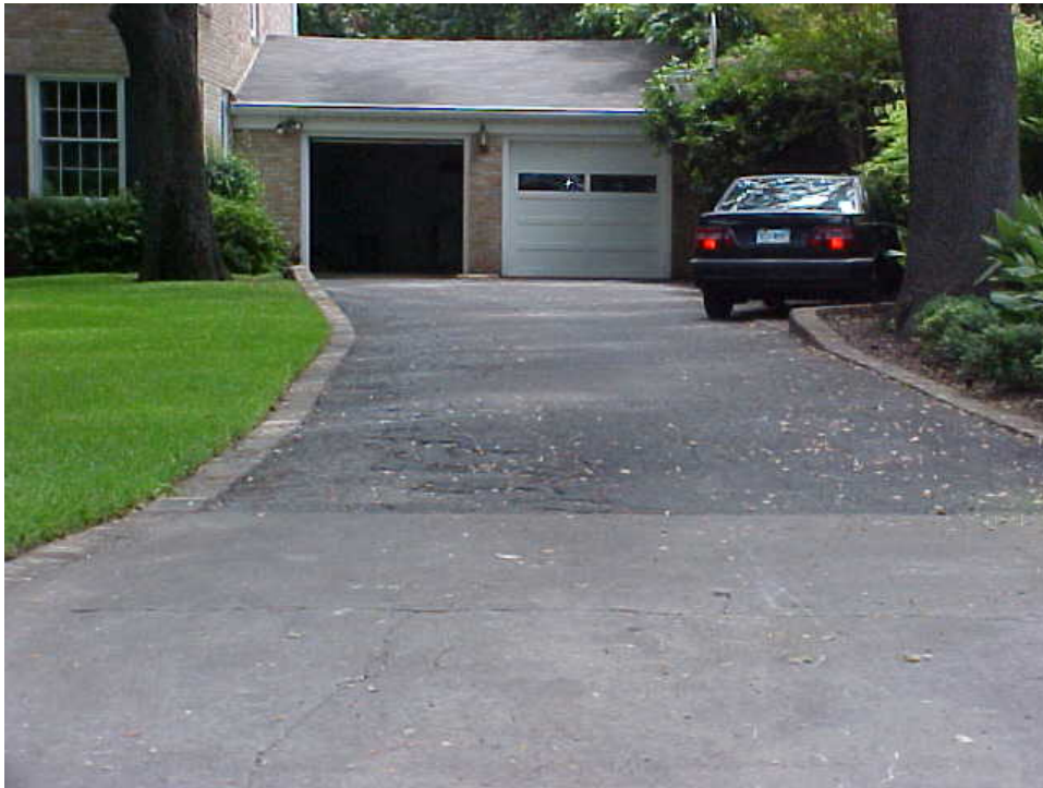
Existing asphalt driveway with the concrete apron.
