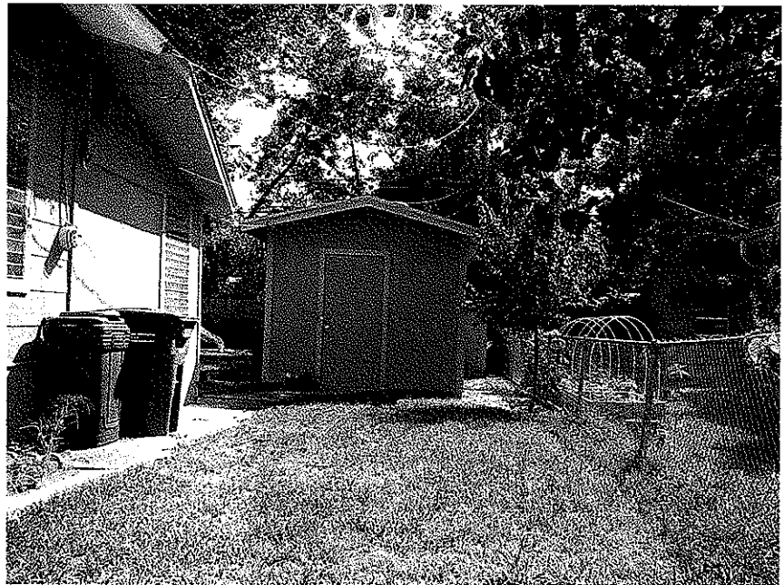
looking at shed from the north
