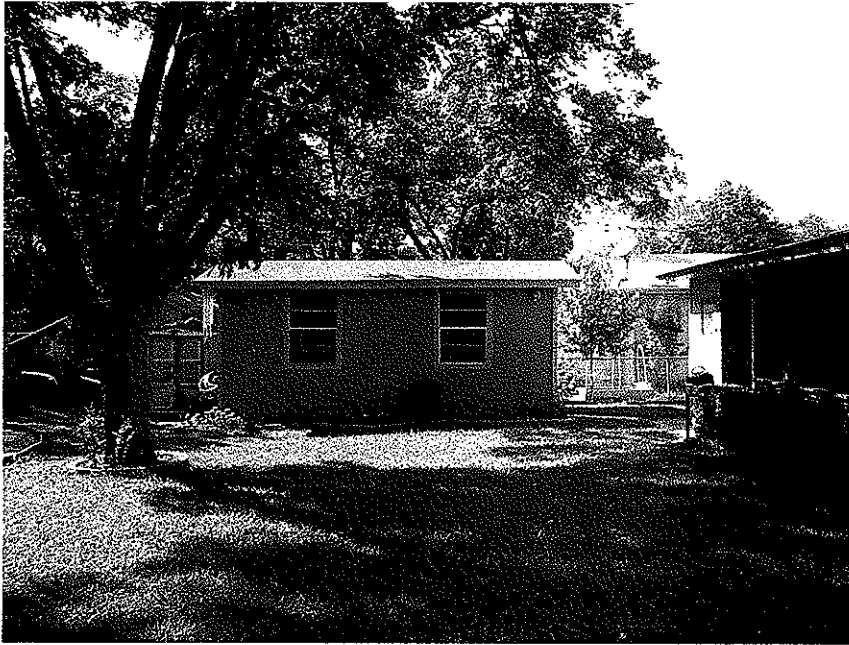
looking at shed from the east
