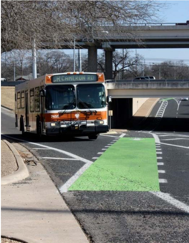
One of the colored lanes installed along Dean Keeton Street at Interstate 35
