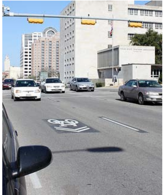
A Shared Lane Marking installed on Guadalupe Street in downtown Austin
