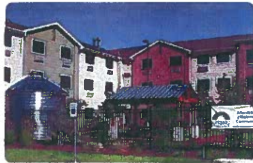
Spring Terrace (renovation of Hearthside Extended Stay Hotel)
