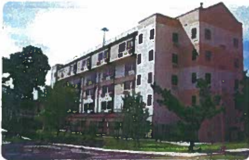
Skyline Terrace (renovation of a former Ramada Inn)
