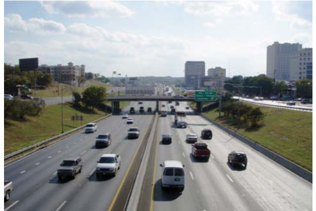
IH 35, completed in the 1970s, created a significant barrier between Downtown and East Austin.
