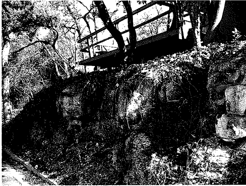
The Existing Front Deck from Alameda
