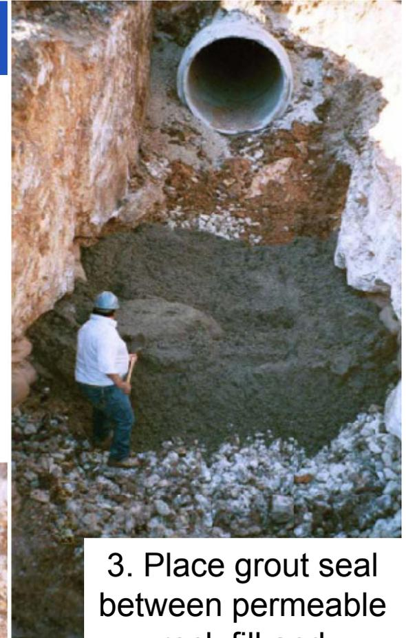
3. Place grout seal between permeable rock fill and wastewater pipe that extends 5 ft above cave roof
