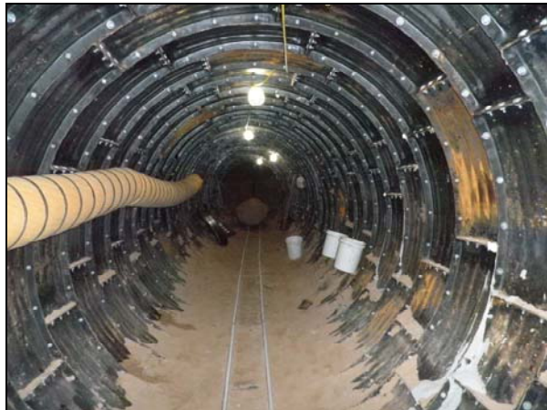
Tunneling operation to install a new 72-inch RCP under the CapMetro Redline as part of the East 4 th /Pedernales stormdrain improvement project.
