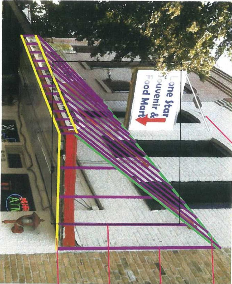
5/16" Suspension Cable attached to sign cabinet and existing wall by eye bolts, anchored and epoxied. Turn buckles installed
