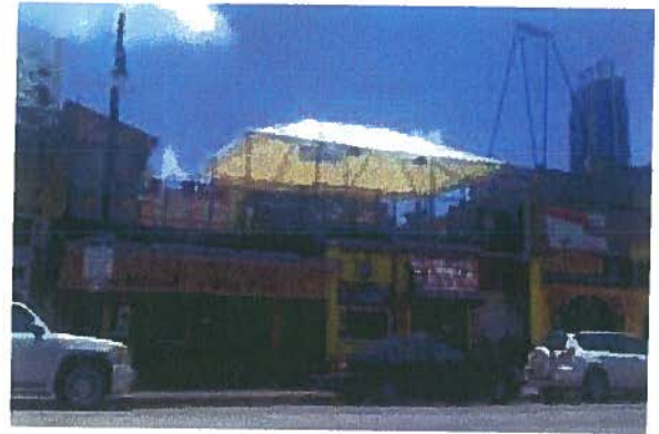
The character of the East 6th Street NRHD has been diminished by ad hoc rooftop additions.
