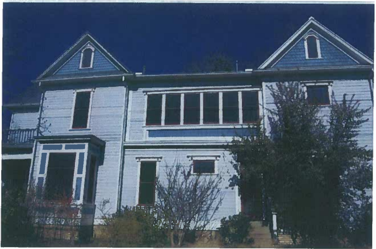
View of the rear of the house, showing the 2001 additions.
