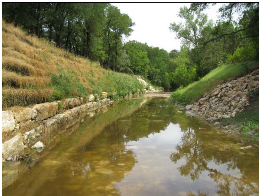
Fort Branch Lott Avenue Channel Rehabilitation
