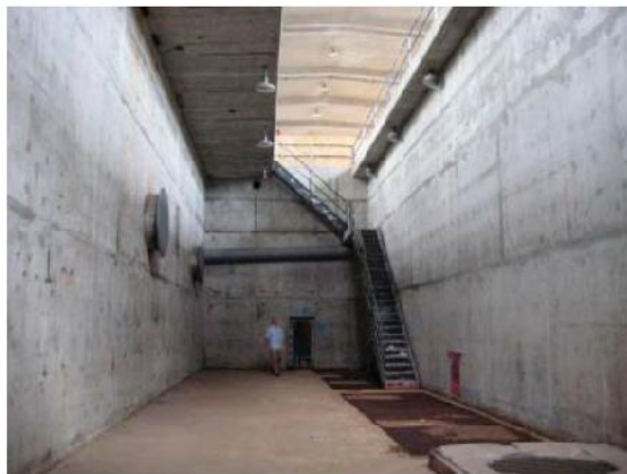
Building A: Pump Room interior space showing stair access.
