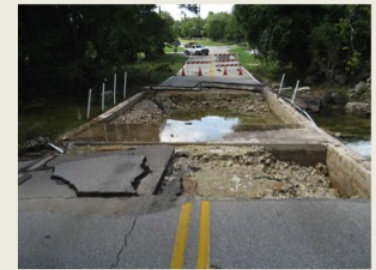
Spicewood Spicewood Springs Road at Bull Creek, September 2010 after flood waters receded.
