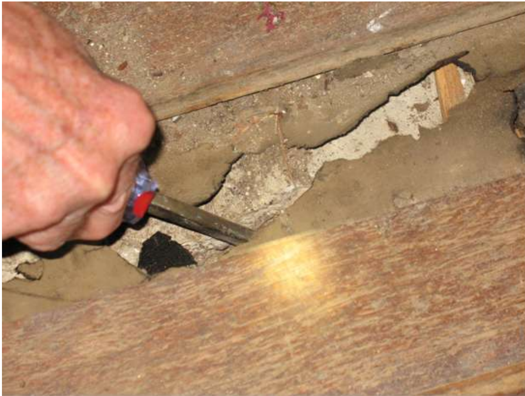
Crack in slab foundation under existing floor boards.
