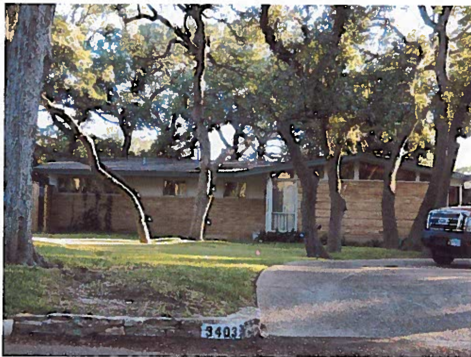
Luedecke Residence, 3403 Foothill Parkway (1952)
