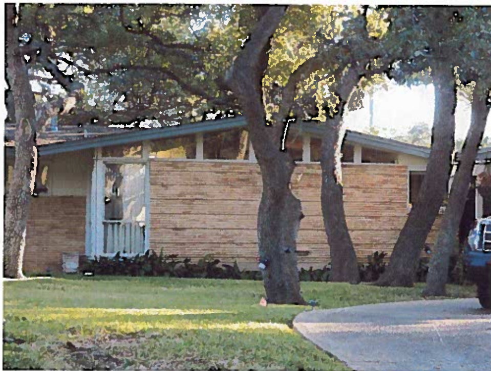
Luedecke Residence, 3403 Foothill Parkway (1952)
