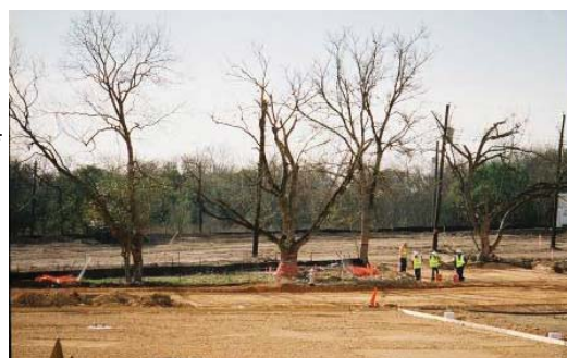
Figure 45 37: Examples of tree preservation during construction.
