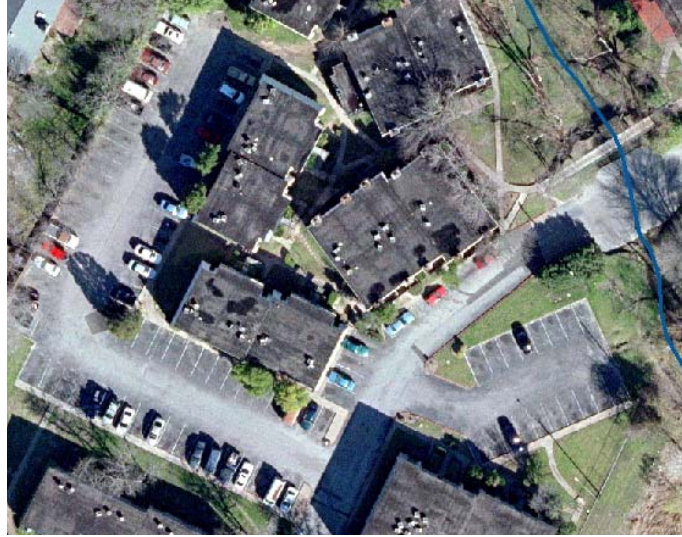
Figure 1. Worn Parking Lot in Austin, Texas.
