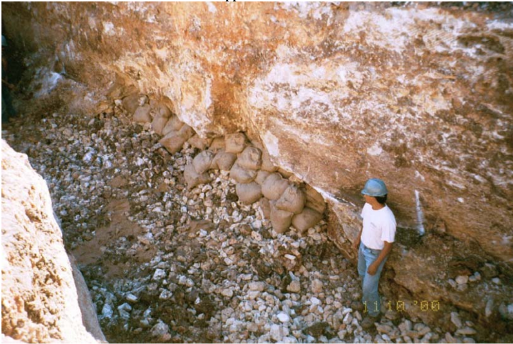
Sand bags placed inside cave opening.
