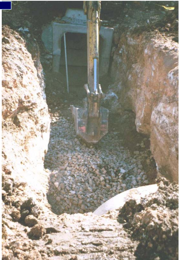
1.8 m (6 ft) diameter RCP stormsewer
