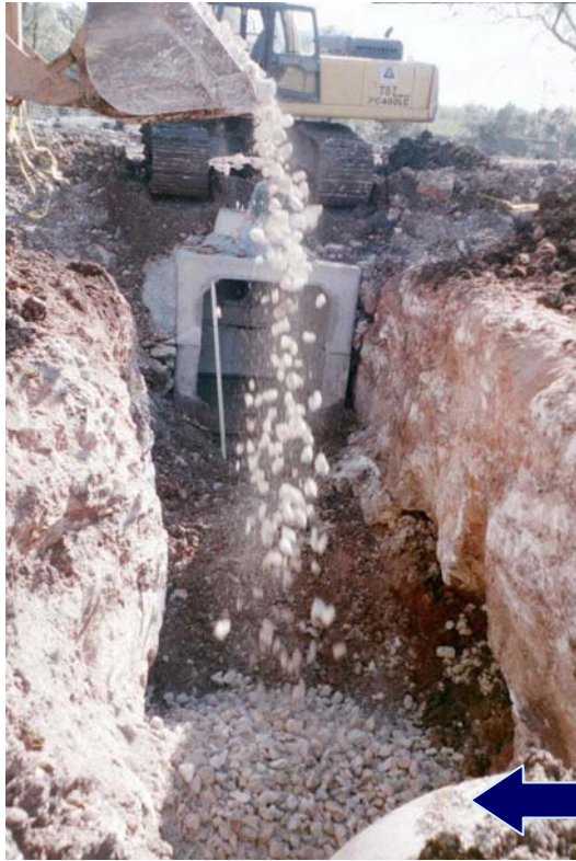
1.8 m (6 ft) diameter RCP stormsewer
