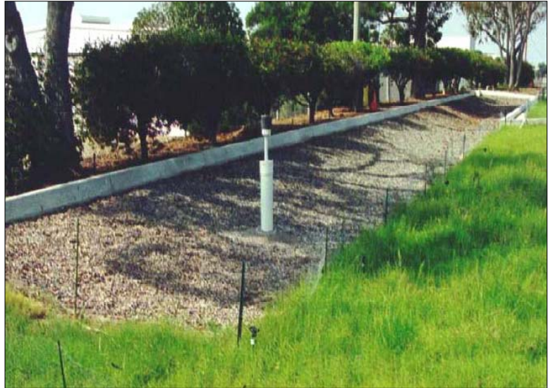
Figure 3 - Infiltration Trench
