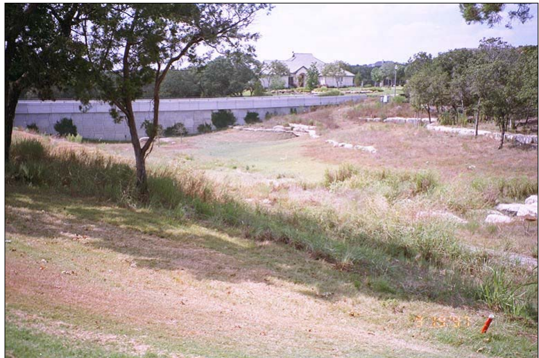
Figure 4 - Extended Detention Pond
