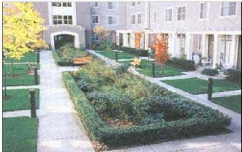
Figure 7 - Bio-Retention System
