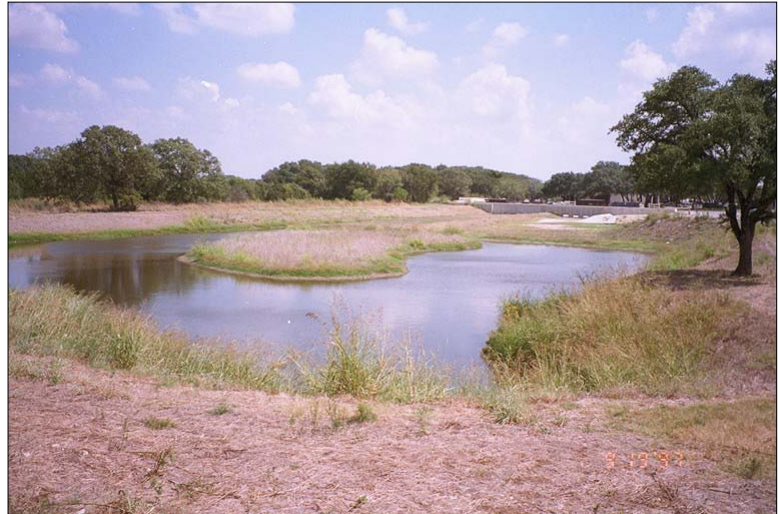
Figure 5 - Wet Detention Pond
