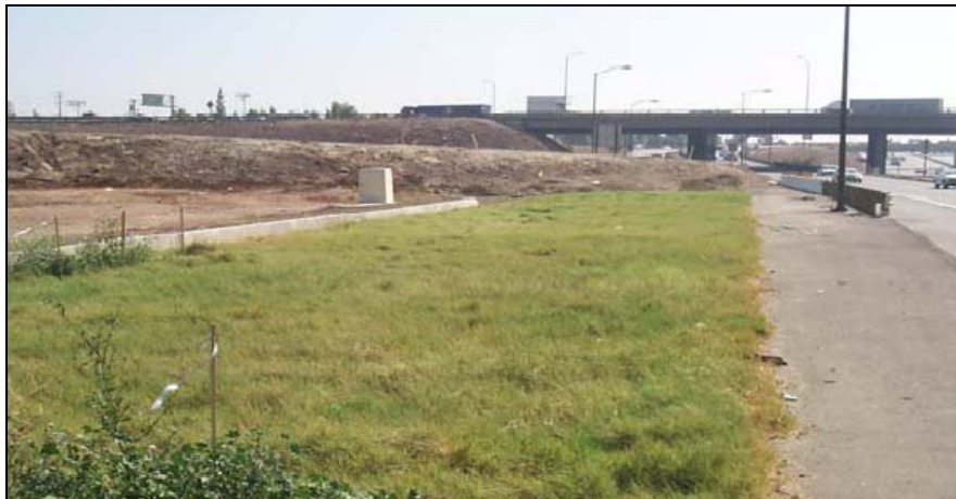
Figure 2 - Vegetative Filter Strip Adjacent to Roadway
