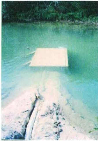
Figure 2: (left) Concrete vault and valve system above Antioch Cave within Onion Creek. (above) Sodium fluorescein dye being poured into the top of the vault.
