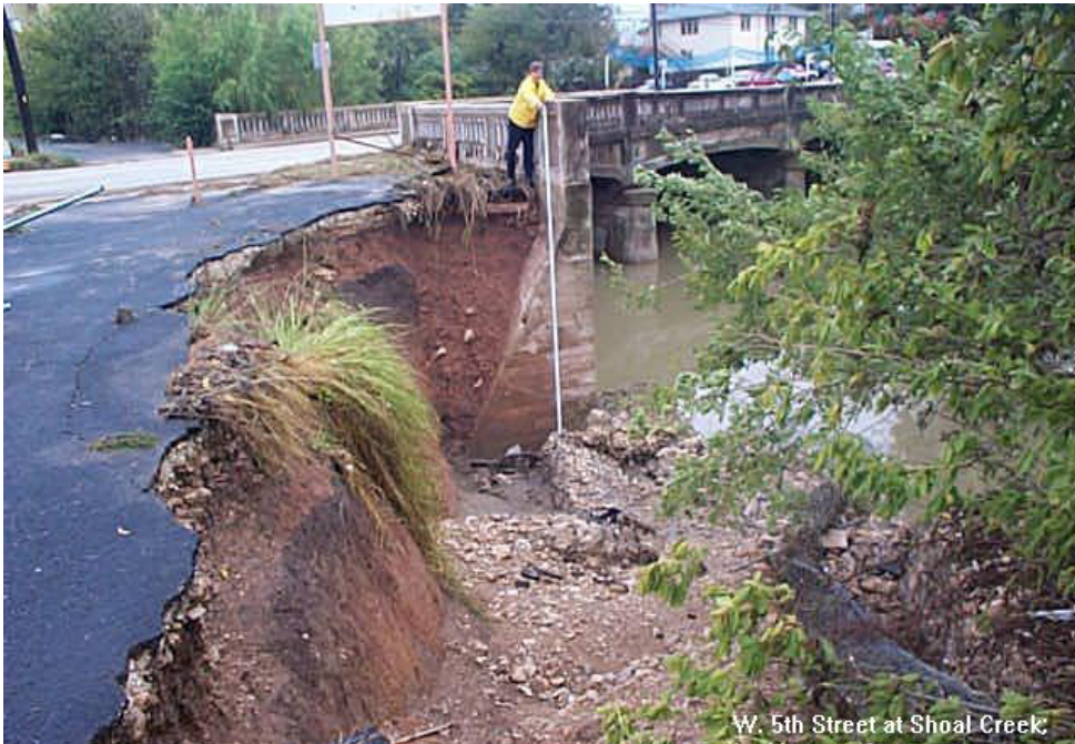
West 5 th Street Bridge at Shoal Creek (looking south) November 16, 2001
