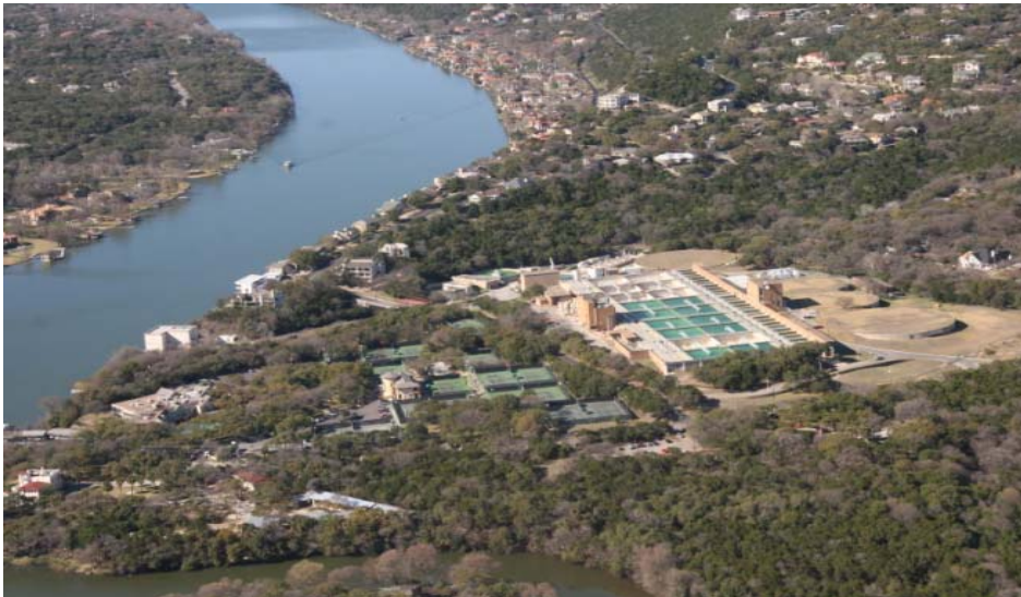
Davis Water Treatment Plant
