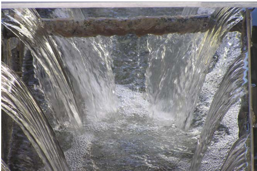
Reclaimed water ready to be used at the cooling tower at Austin Energy's Sand Hill Energy Center – a natural gas fired electric generation plant near the South Austin Regional Treatment Plant
