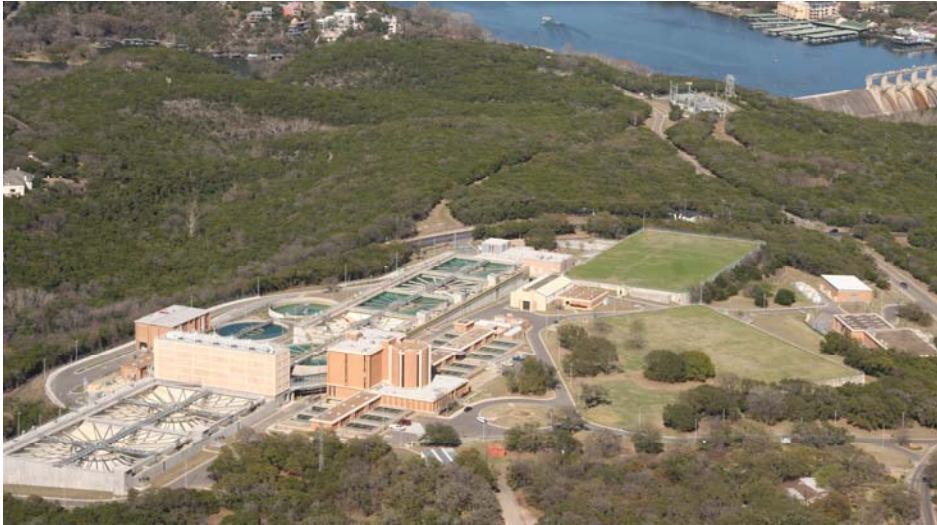
Ullrich Water Treatment Plant
