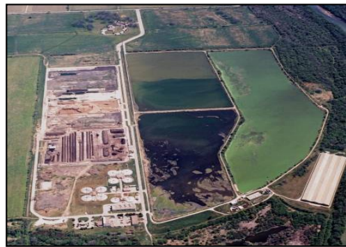
The Hornsby Bend Biosolids Management Plant
