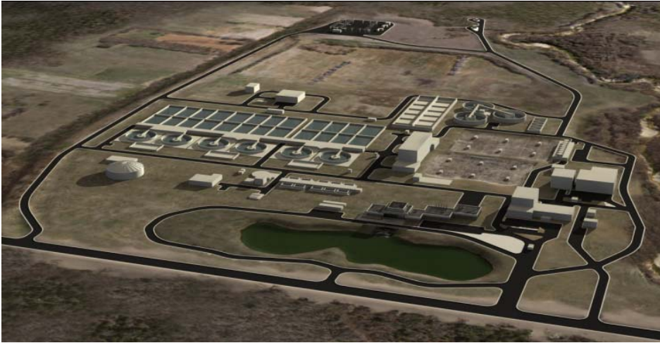
Walnut Creek Wastewater Treatment Plant
