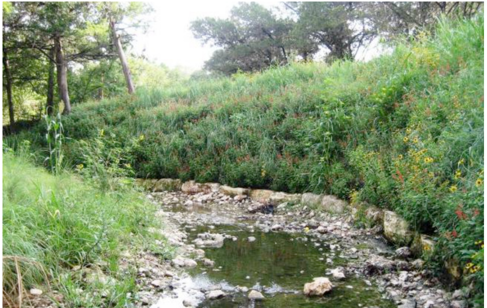
Example of a streambank restoration project, using limestone and native plants.
