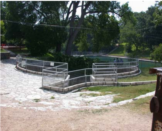
A) Protective Berm at Base of Fence
