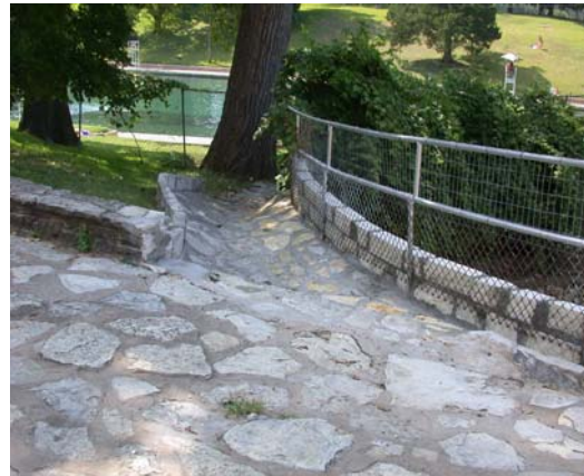
B) Reconstructed Swale
