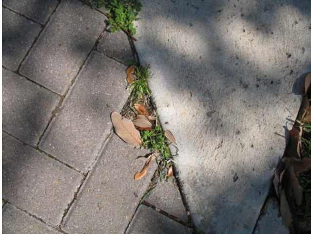
Corner brick missing (on path near snake's head)
