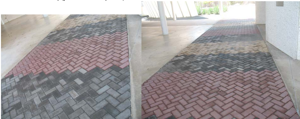
Under the overhang the bricks are different colors, likely due to moisture under the bricks and/or mold
