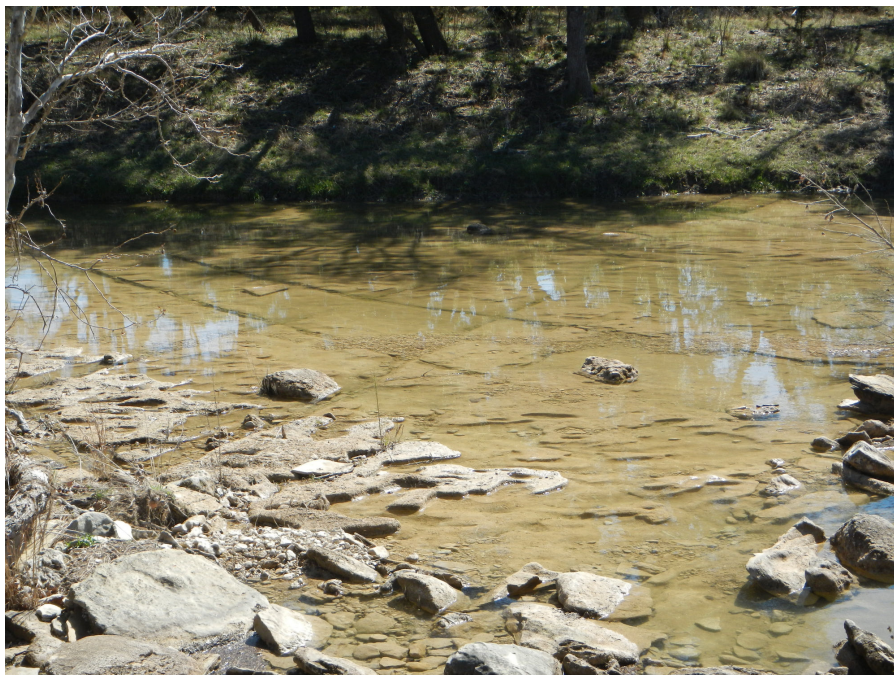
Photo 4. Limestone bedrock with prominent fractures trending N48E and N32W which are visible on aerial imagery in Photo 5.
