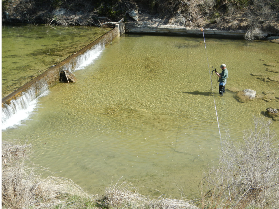
Photo 3. Site “On 3” showing limestone bedrock channel bottom and bank. The check dam is approximately 4 ft high.
