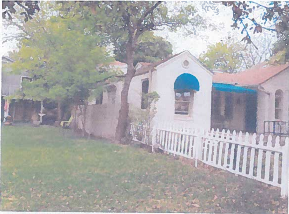
Northwest corner of the house.
