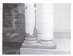
Deteriorated wood porch elements can be repaired in place with epoxy consolidants and fillers.
