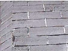
Sandblasting and other abrasive cleaning methods can permenantly damage exterior building materials. Clean masonry surfaces with the gentlest method possible, such as low pressure water and detergents, using natural bristle brushes.
