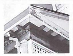
Damaged exterior wall materials can be repaired or replaced in kind, as in this example of a replaced facia board.
