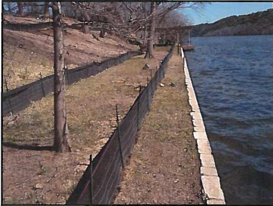
Photo 1. View of the shoreline at 901 River Road
