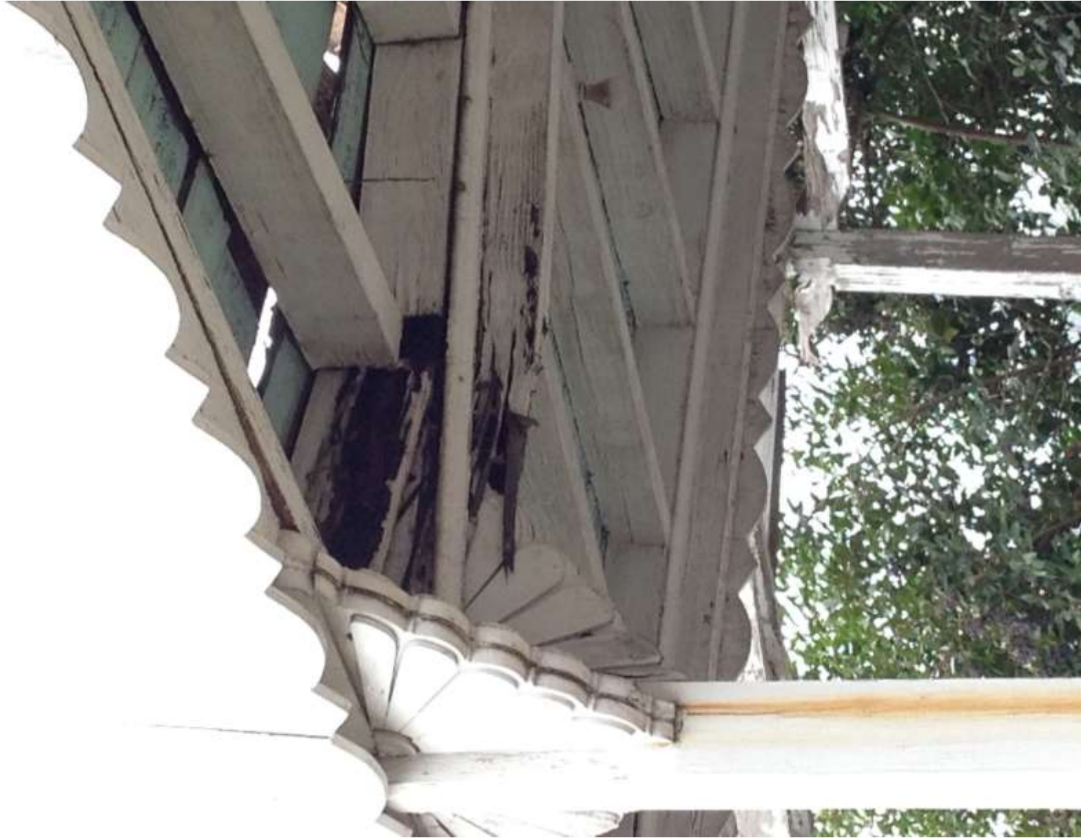
Main beam of second floor has failed.
