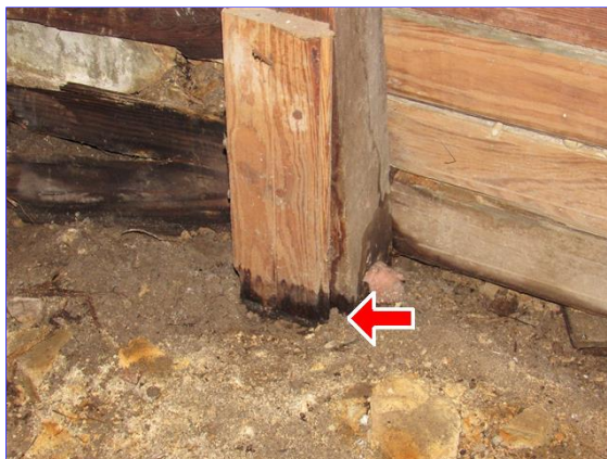
Deteriorated post
