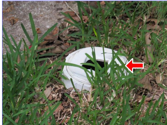
Damaged clean-out cap
