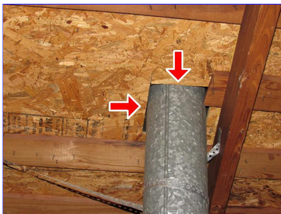
Insufficient clearance from roof decking
