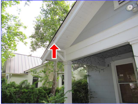
Location of missing drip-edge
