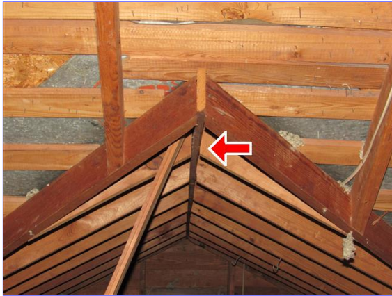
Undersized ridge beam
