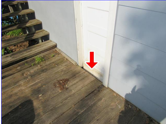
Deck higher than the Storage Entry
