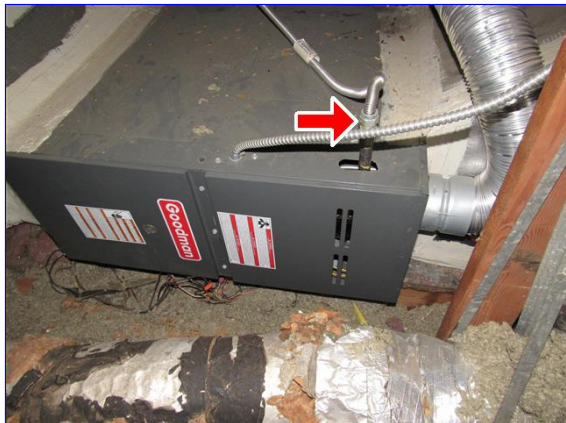
Location of missing sediment trap
