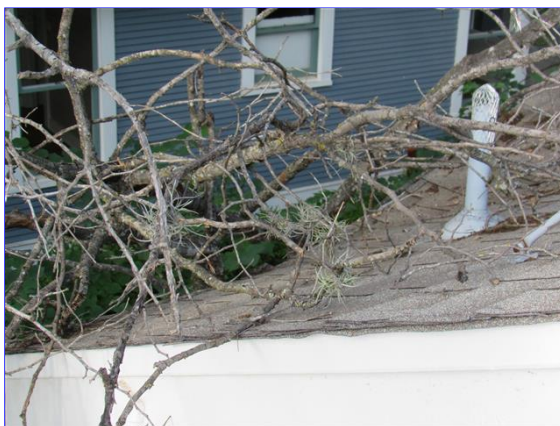
Tree limbs in contact with the roof
