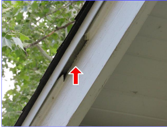
Location of missing drip-edge
