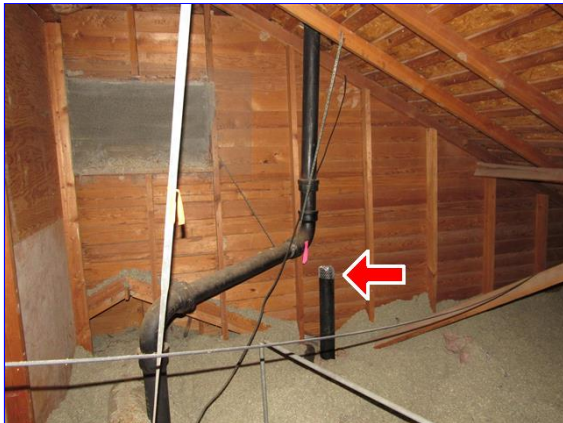
Improper vent termination
