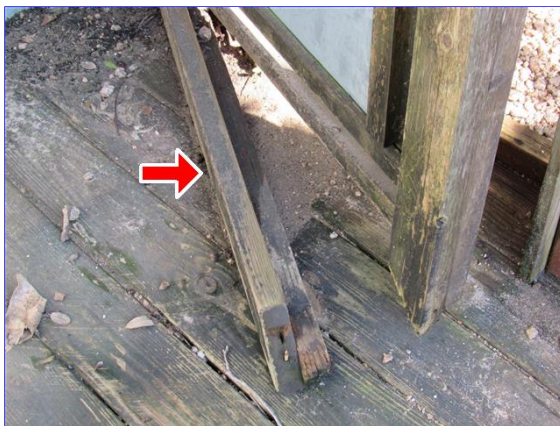
Damaged rear entry gate
