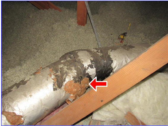
Example of failed ducting
