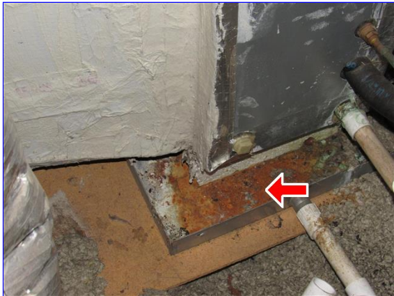
Rust at secondary drain pan
