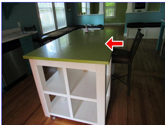
Island missing an electrical receptacle
