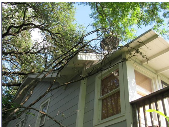
Tree limbs in contact with the roof
