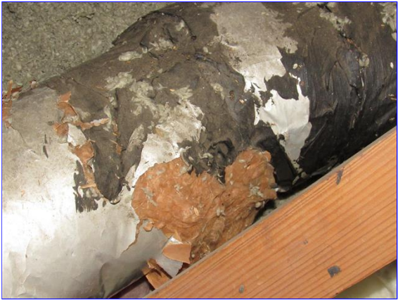
Example of failed ducting
