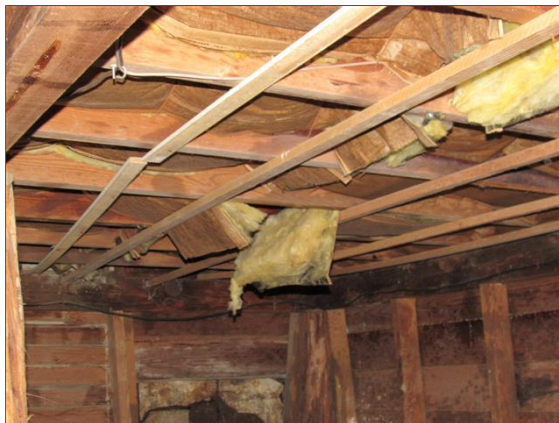
Example of loose flooring insulation
