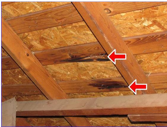
Evidence of moisture penetration
