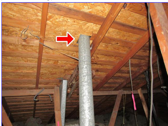
Insufficient clearance from roof decking
