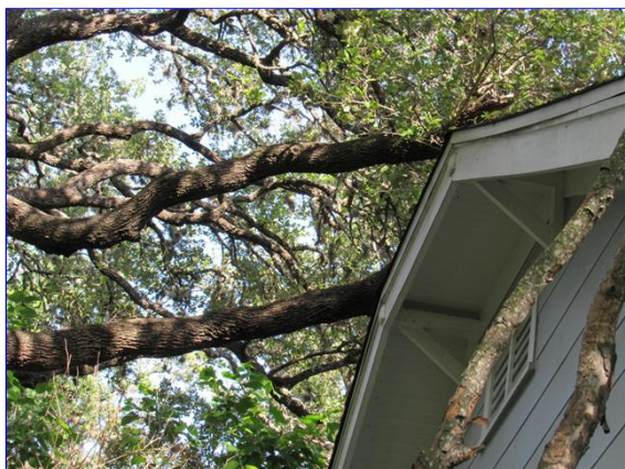
Tree limbs in contact with the roof
