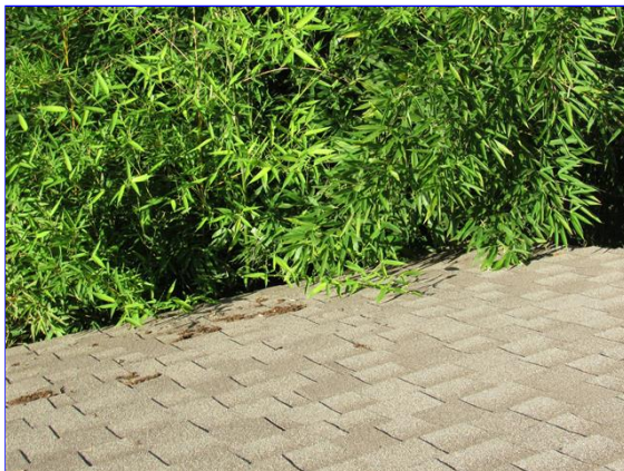
Tree limbs in contact with the roof
