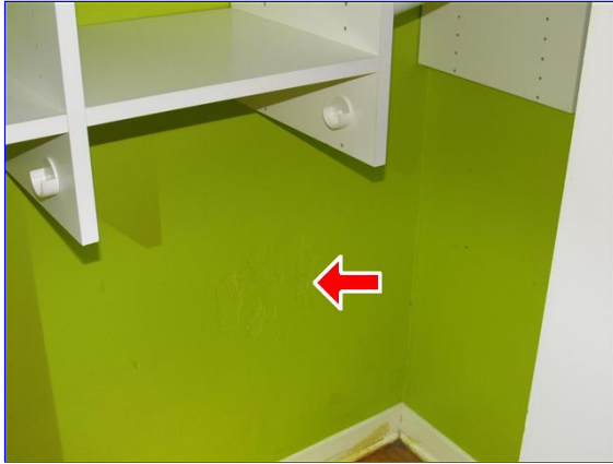
Location of termite damage
