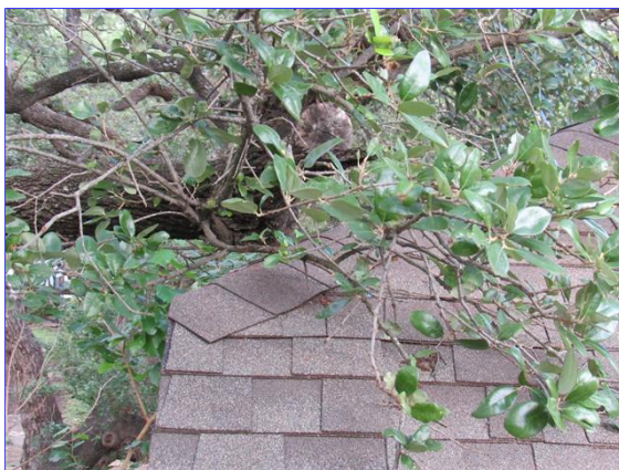
Tree limbs in contact with the roof
