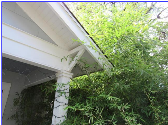
Tree limbs in contact with the roof
