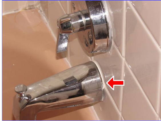
Nozzle gapped at wall
