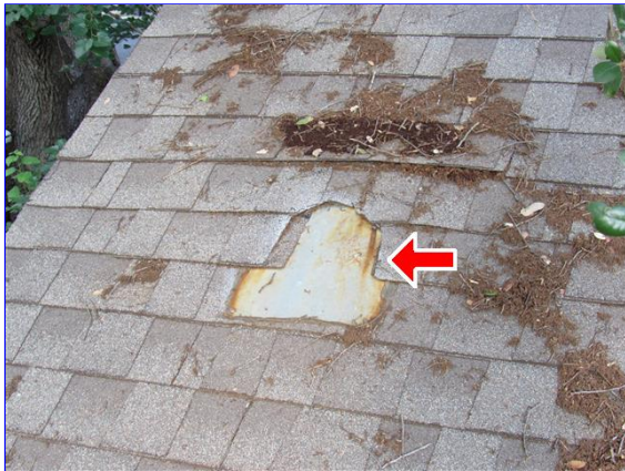
Flashed previous vent penetration
