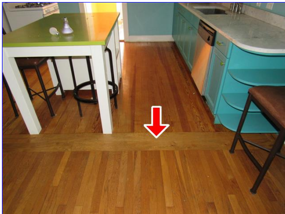
Location of loose/noisy flooring
