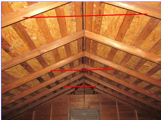
Location of missing collar ties
