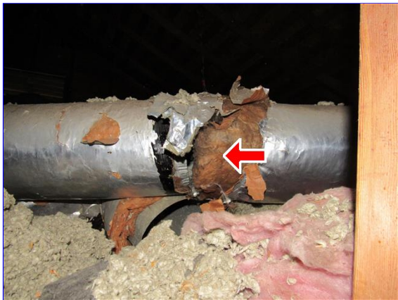
Example of failed ducting
