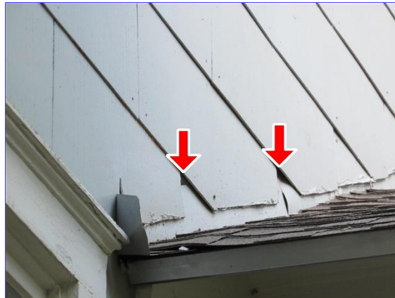
Gapped cladding at flashing
