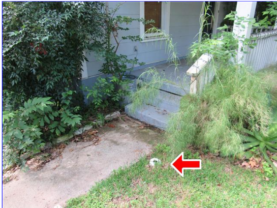
Damaged clean-out cap
