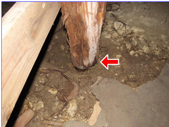
Example of post deterioration
