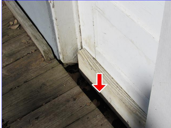
Deck higher than the Storage Entry
