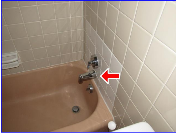
Nozzle gapped at wall
