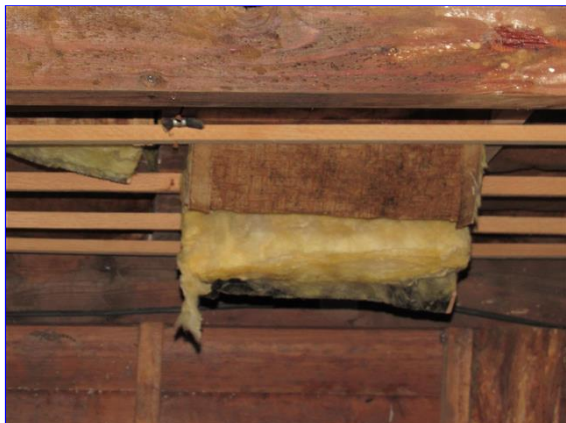
Example of loose flooring insulation
