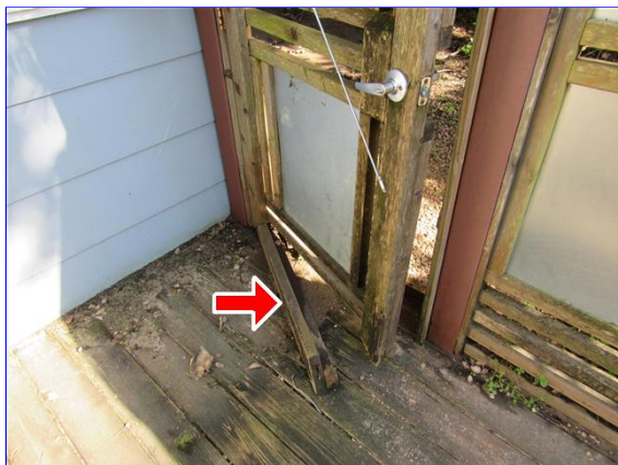
Damaged rear entry gate
