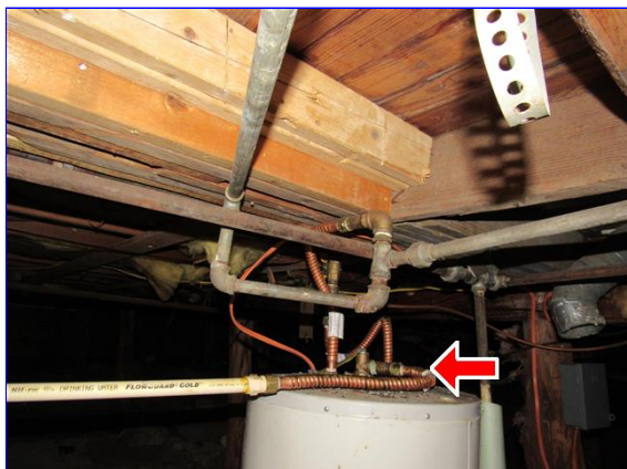
Non-insulated water lines
