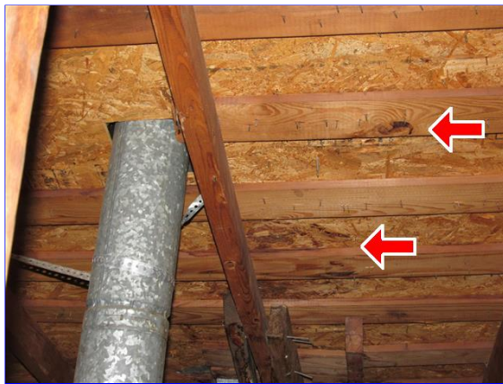
Evidence of moisture penetration
