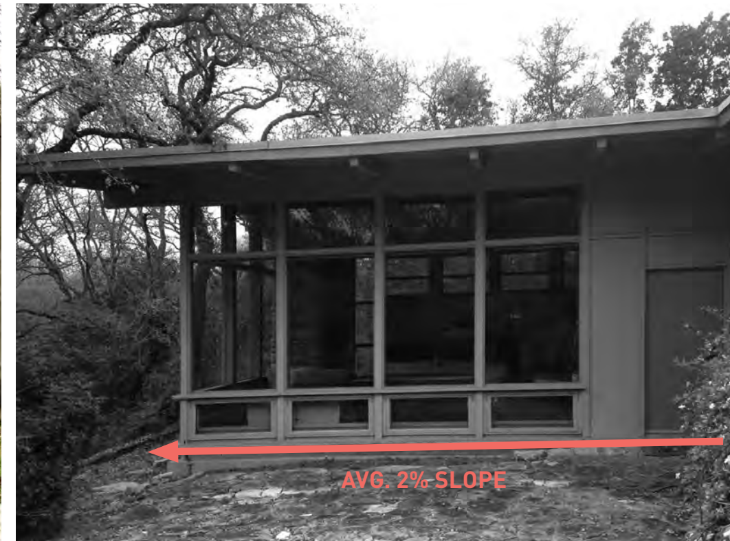
Entry. Portion with the most severe slab displacement (12" out of level on the east end at a slope of 1:51 - anything over 1:20 is considered a ramp, not occupiable slab).
