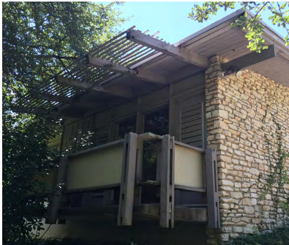
Master Bedroom deck is significantly rotting.
