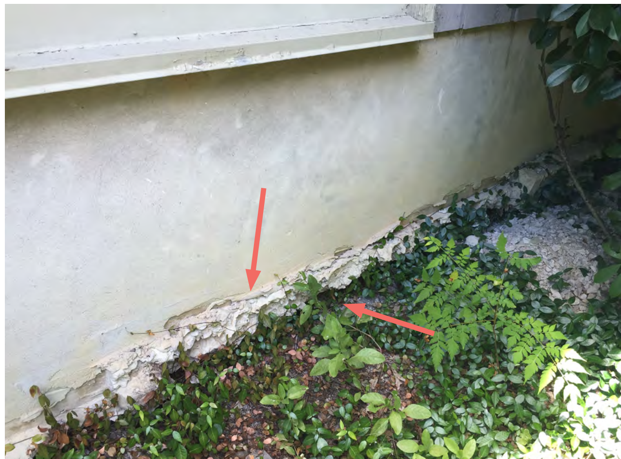
Foundation settlement on east face of Bedroom wing. A severe (6") gap between the foundation and top of soil is evidence of significant erosion below the foundation.
