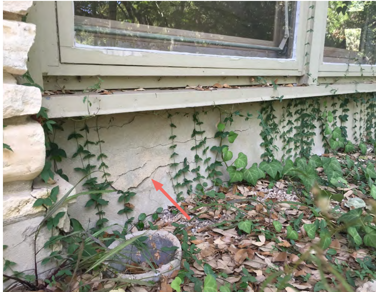
Numerous and large cracks as a result of foundation settlement on east face of Living Room.
