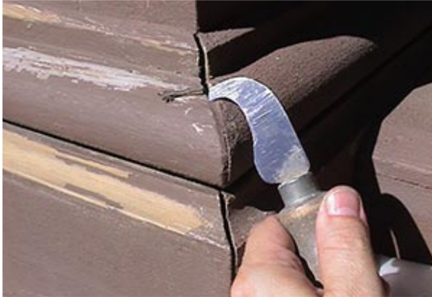
Cracks and unpainted wood on porch elements can lead to decay due to water seepage. Proper caulking and painting can help preserve these elements.-- http://www.nps.gov/tps/how-to-preserve/briefs/45-wooden-porches.htm
