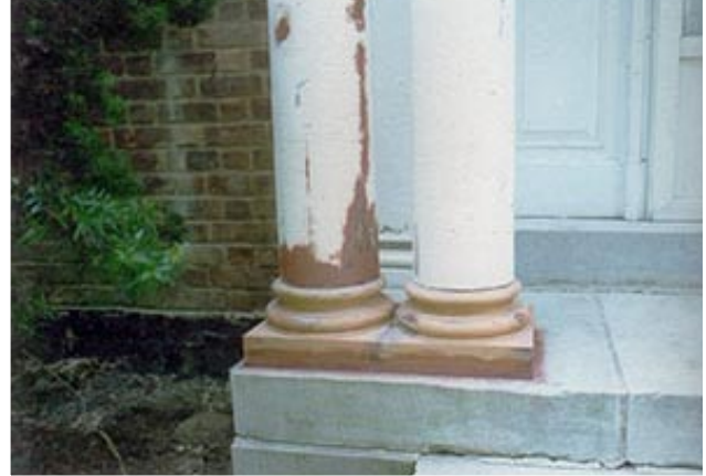
Deteriorated wood porch elements can be repaired in place with epoxy consolidants and fillers. -- http://www.nps.gov/tps/how-to-preserve/briefs/45-wooden-porches.htm
