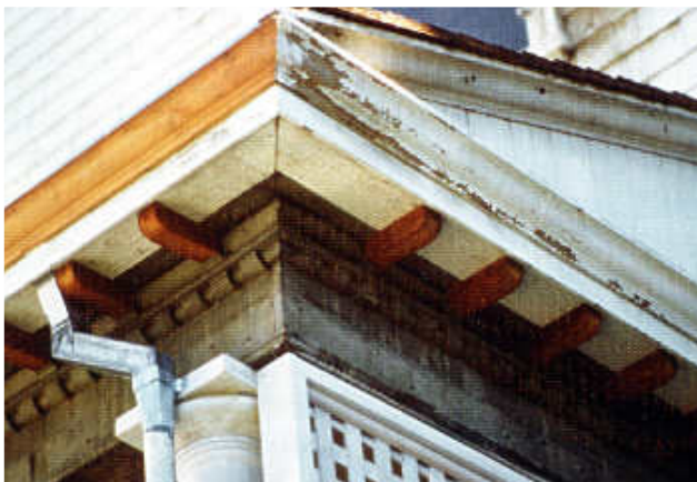
Damaged exterior wall materials can be repaired or replaced in kind, as in this example of a replaced fascia board. -- http://www.cr.nps.gov/hps/tps/standguide/preserve/preserve_wood.htm
