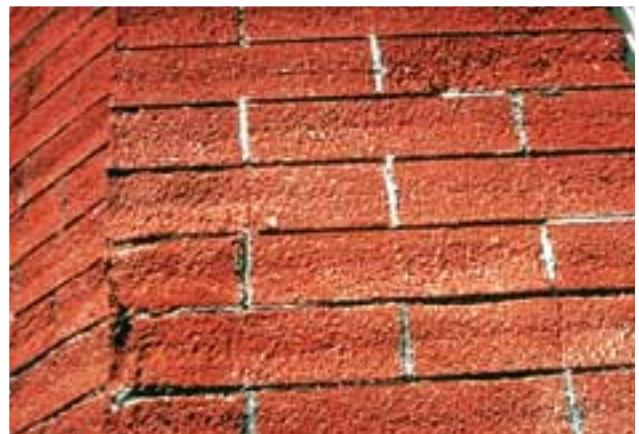
Sandblasting and other abrasive cleaning methods can permanently damage exterior building materials. Clean masonry surfaces with the gentlest method possible, such as low pressure water and detergents, using natural bristle brushes.-- http://www.cr.nps.gov/hps/tps/standguide/rehab/rehab_masonry.htm
