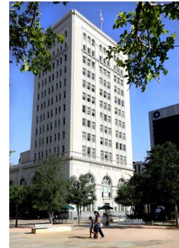
Right: DAO = San Antonio Municipal Plaza Building
