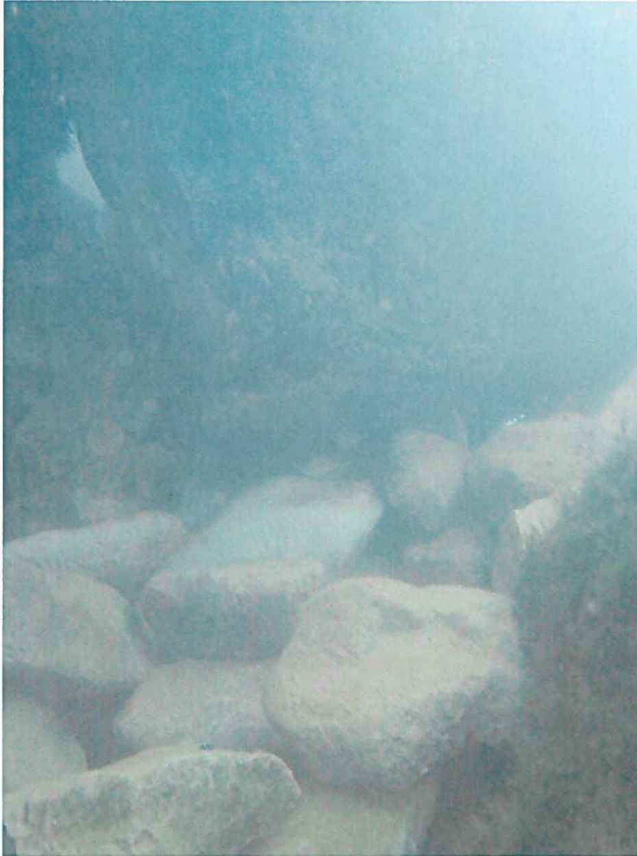
Figure 2. Rock fill (bottom of photo) placed below boulder (top) that fell into Barton Springs Pool to prevent swimmers from entering the void under the boulder.
