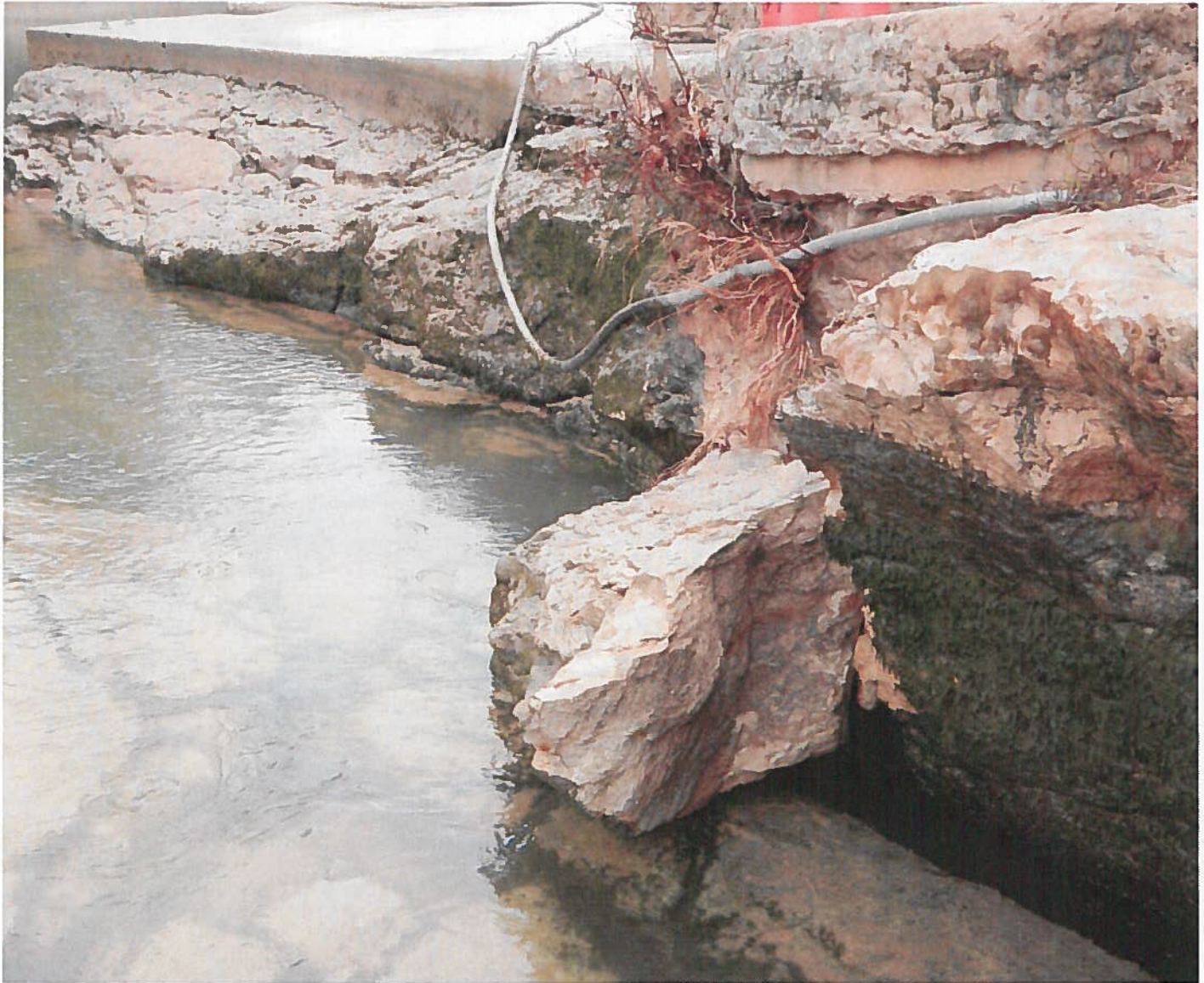
Figure 1. View of boulder that calved from the rock face in Barton Springs Pool during a post-flood drawdown in early November, 2016.
