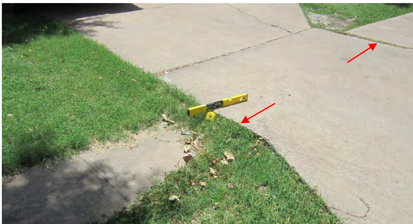
Figure 4. Sidewalk Faults at Driveway Interfaces
