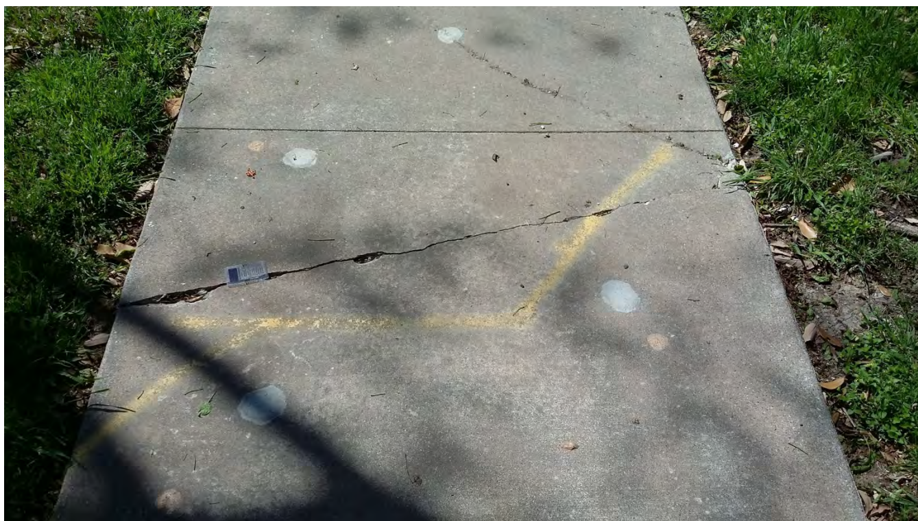
Figure 2. Cracking Ex. 2: Moderate
