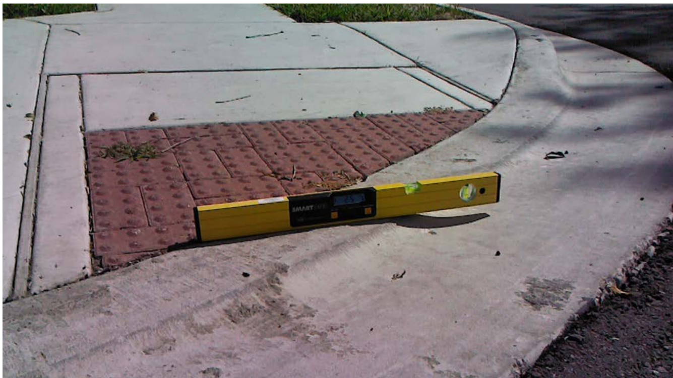
Figure 8. Curb Lip Fault (Formed/Constructed)
