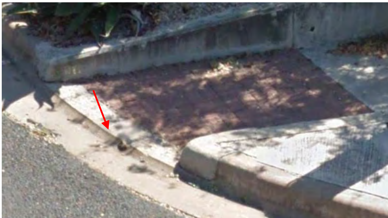
Figure 7. Curb Lip Fault (Sawed)
