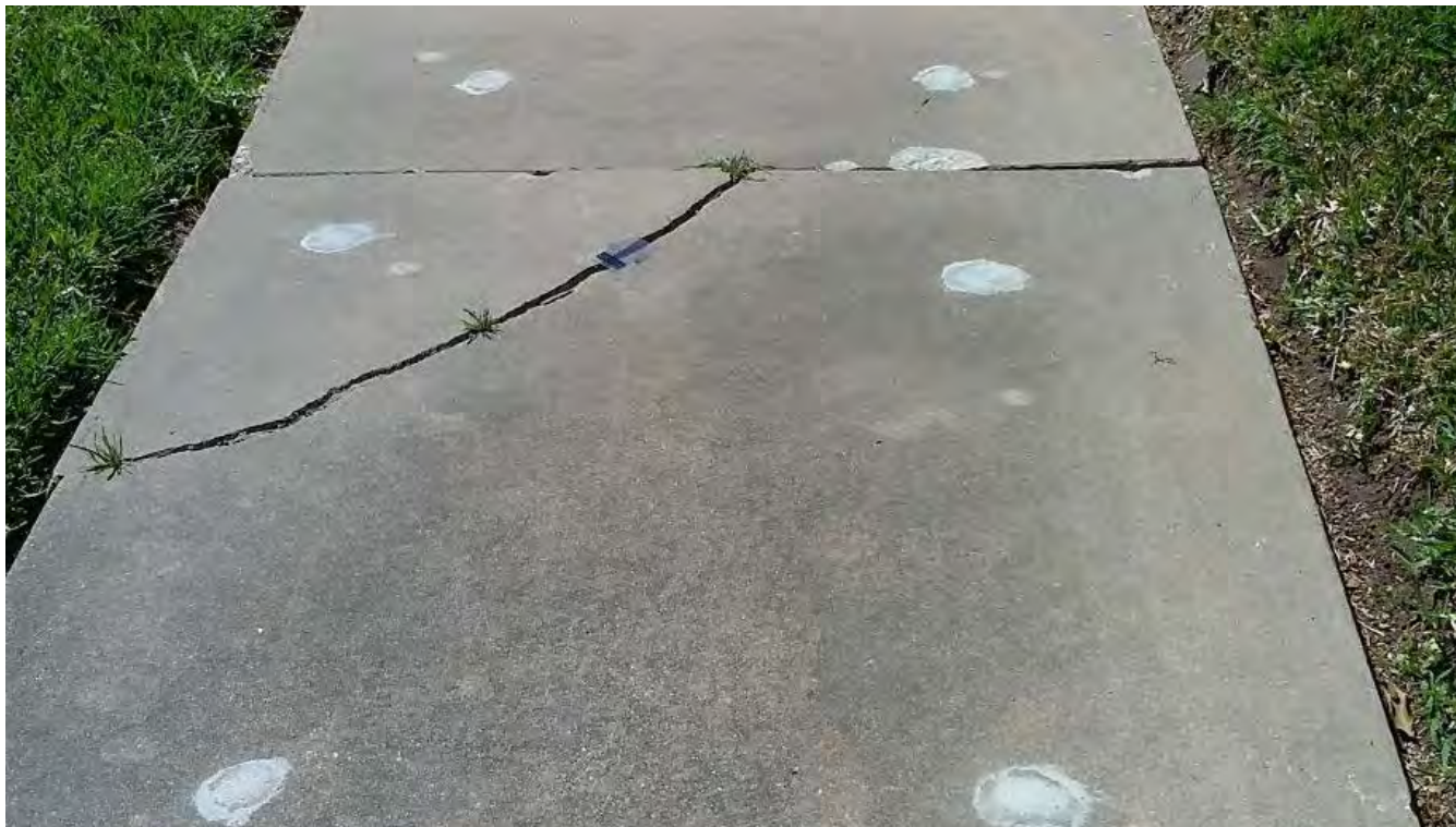
Figure 3. Cracking Ex. 3: Moderate
