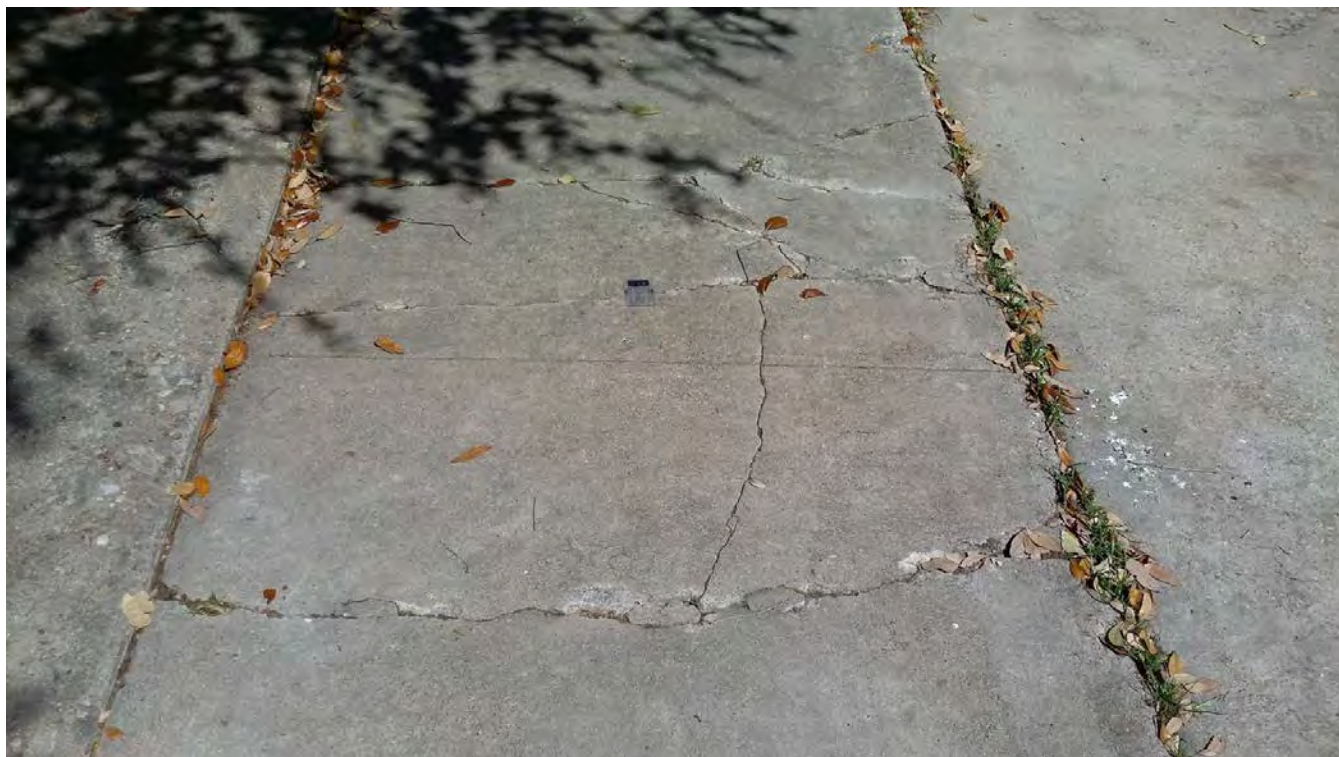
Figure 1. Cracking Ex. 1: Severe
