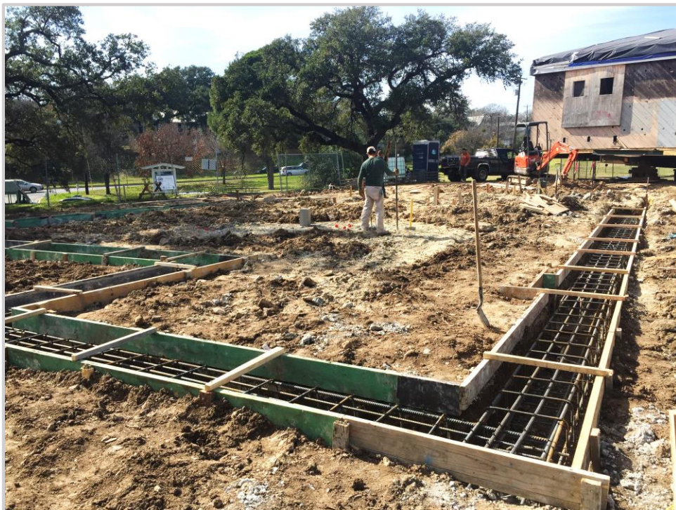
After the piers were cured, the grade beam was formed.
