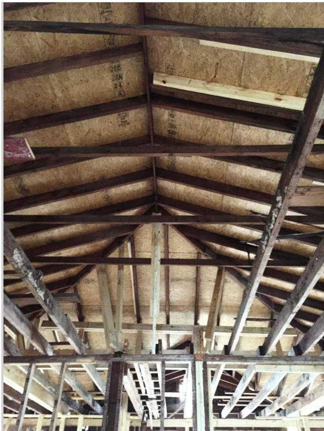
Temporary roof structure was added above the ceiling joists, the existing roof decking was removed, and deteriorated rafters were sistered or replaced as necessary.
