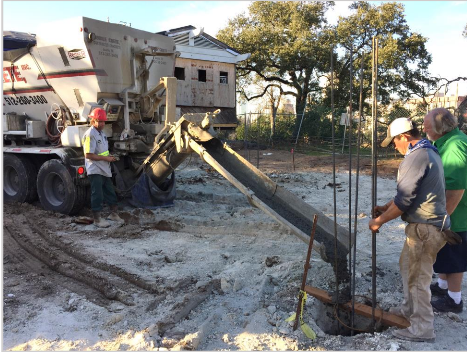
Reinforcing steel was assembled and placed and concrete was poured to form the below-grade foundation piers.
