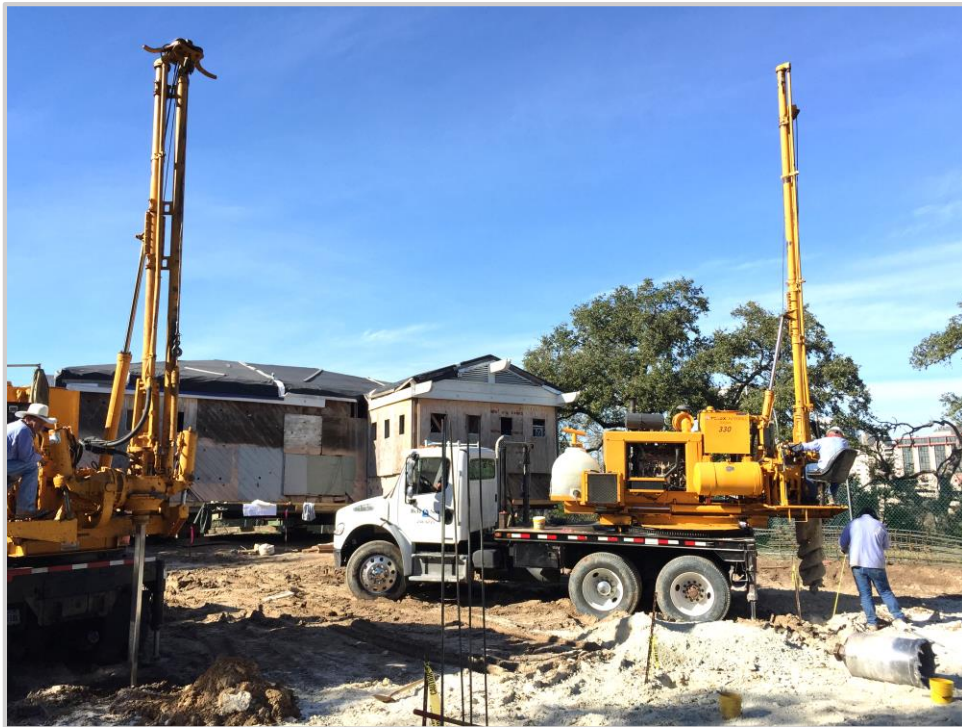
Holes for twenty piers were drilled to bedrock.
