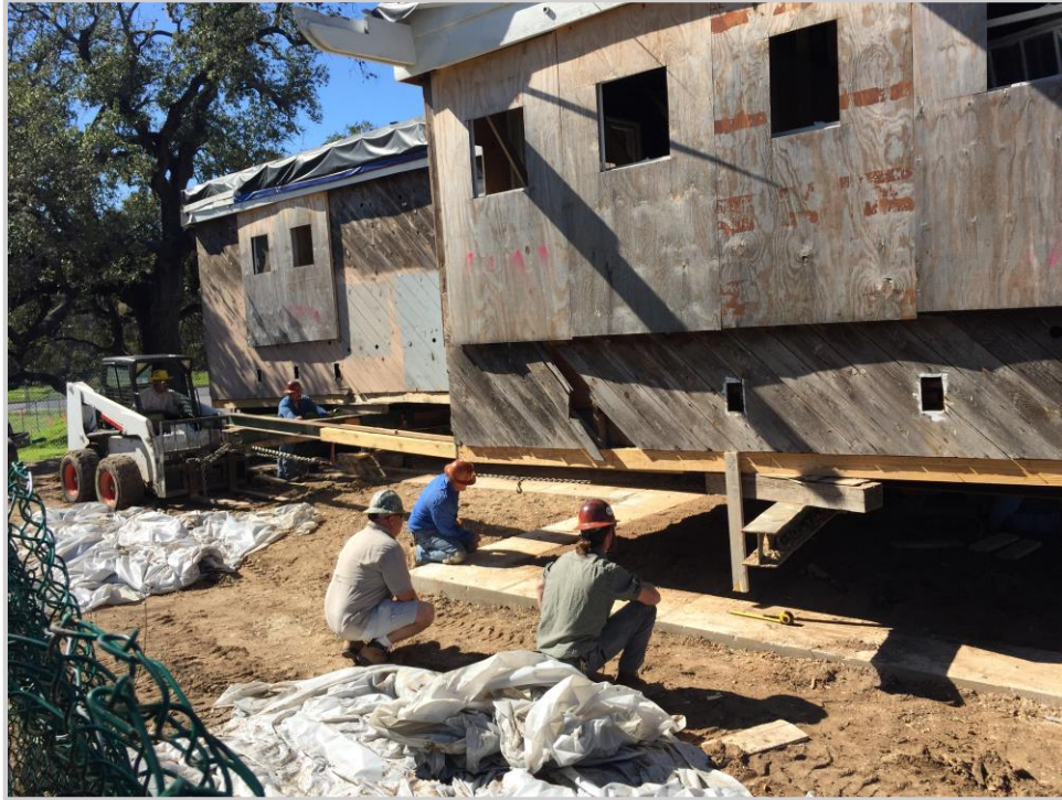
The house was carefully moved into place over the grade beam, to align with the landscape features.
