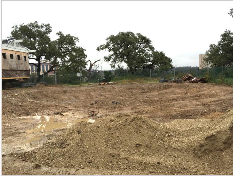
The preexisting foundation, from the 1990s, was fully removed from the site.
