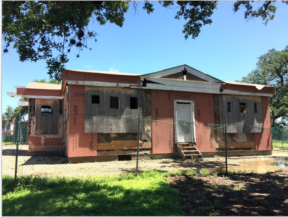
The new rook decking was sheathed with a roll roofing and openings and deteriorated areas of the exterior walls were patched over.
