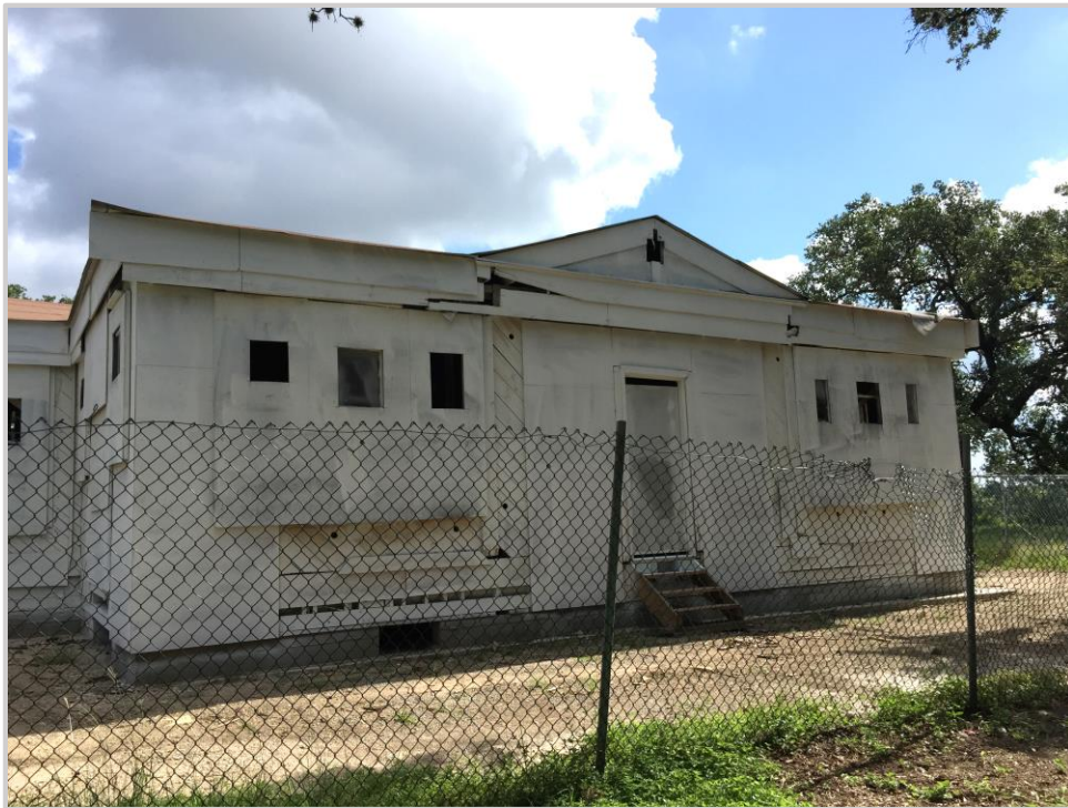
Finally, the exterior of the house has been painted in order to protect the wood and exterior sheathing from additional deterioration.
