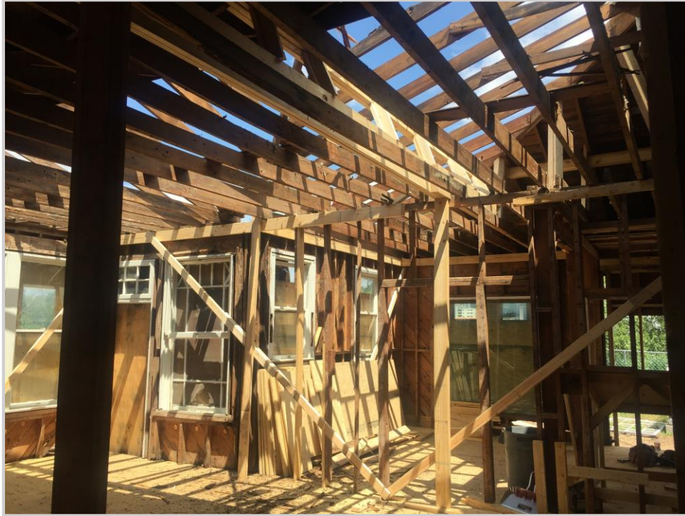
Temporary roof structure was added above the ceiling joists, the existing roof decking was removed, and deteriorated rafters were sistered or replaced as necessary.
