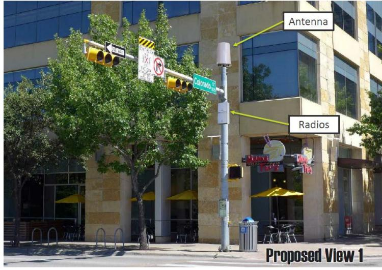
Integrated Antenna & Un-shrouded Radio Module
