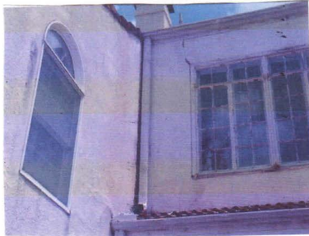
Damaged Exterior Stucco
