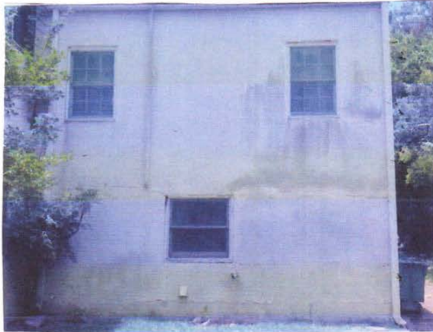
Damaged Exterior Stucco
