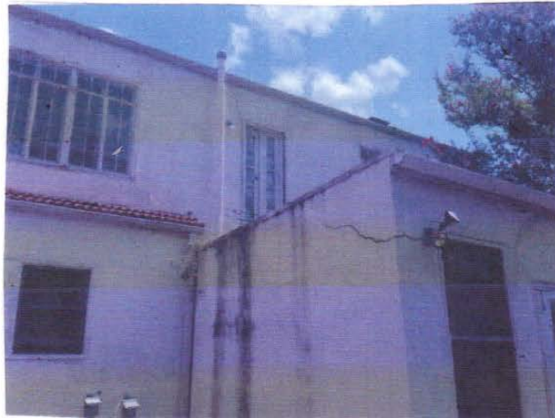
Damaged Exterior Stucco
