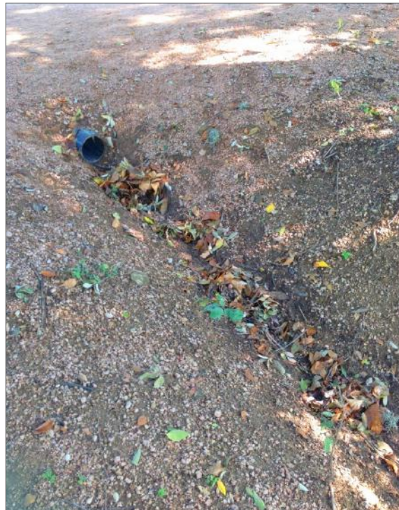
Figure 2.52: Rill erosion often occurs where culverts carry water under the Trail without armoring below.
