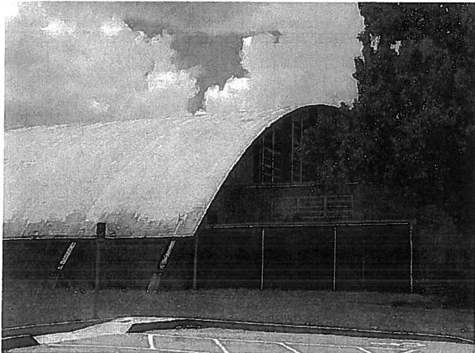
Gymnasium (1961), TSD East Campus
