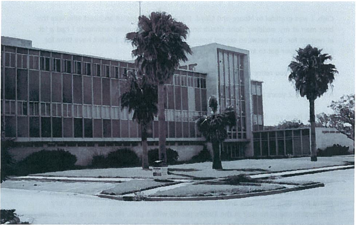
Calhoun County Court House, Port Lavaca, Texas Designed by Rustay & Martin (1959)
