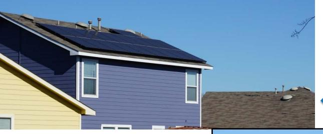
Bunched vents permit solar installation
