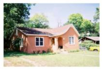
Guideline 1.3: Roofs should be simple in form, either gabled or hipped, with low to moderate pitch (5 or 7:12 is common). Typical roofing materials include metal and tabbed composition shingles.
