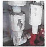
Figure 18: Parking Ops Hydronic Pump and Piping
