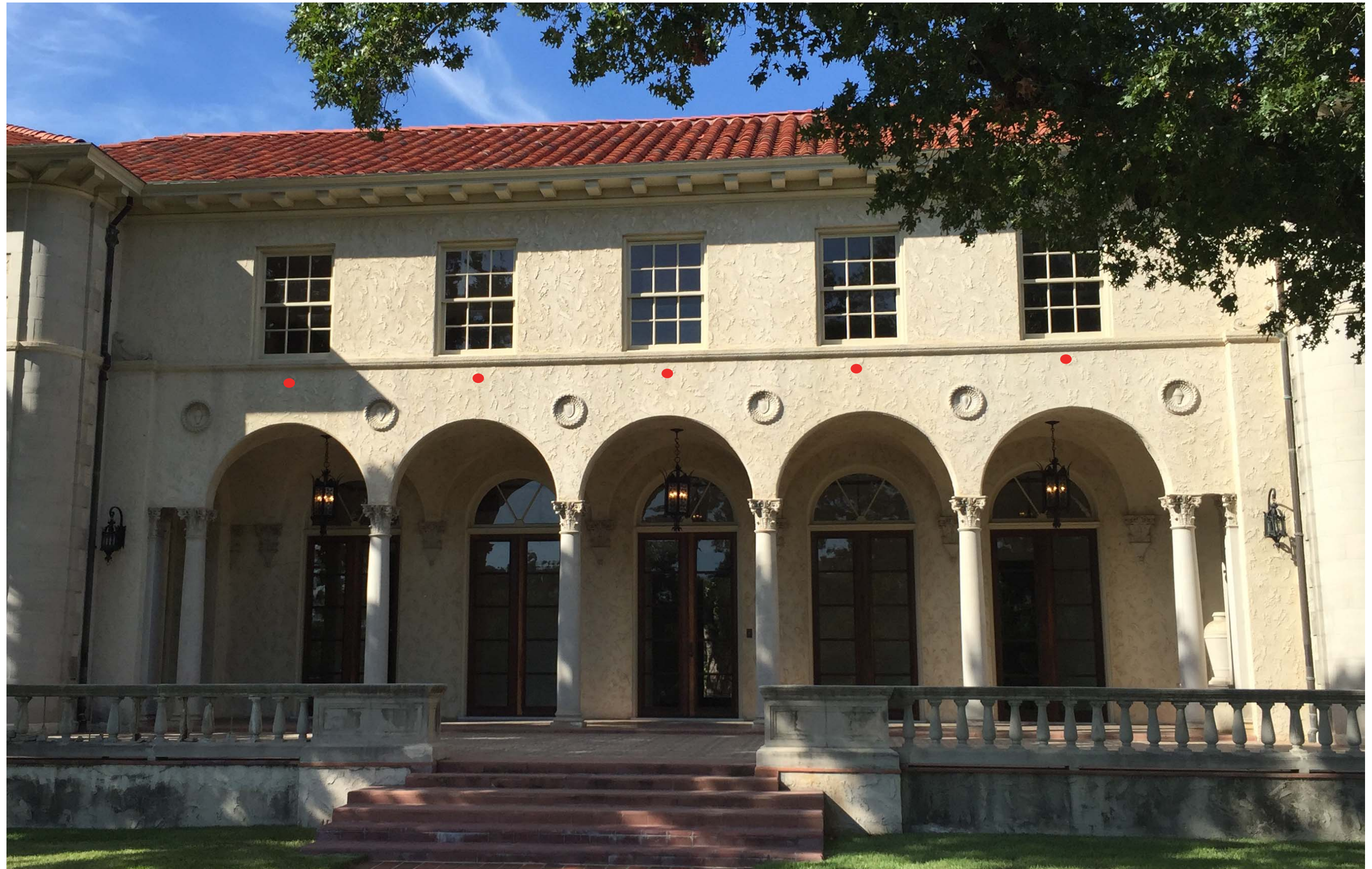
MANSION - CANOPY ADDTION AT SOUTH TERRACE - WALL BRACING CONNECTION LOCATIONS
