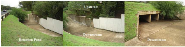
Figure 1a Detention Pond-Type 1 with stepped rectangular weir for flow control (Courtesy: City of Austin, TX)
