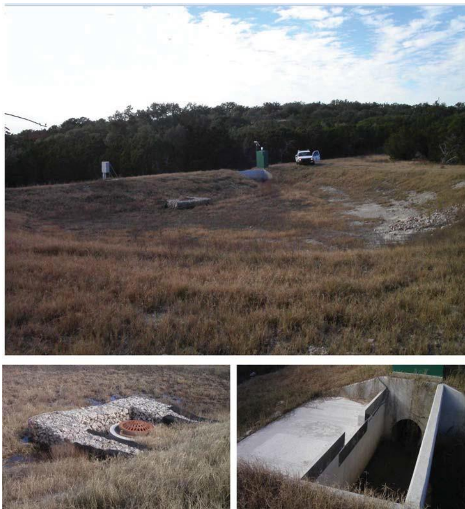
Fig. 1. Retention irrigation system (reprinted with permission from the American Legal Publishing Corporation)
